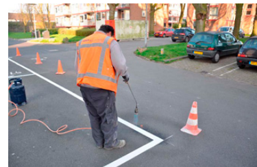
Figuur 4: Thermoplast overlay [6]
