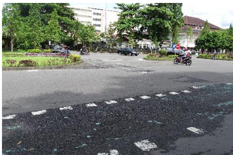
Figure 31 - State 3 - asphalt (Rough with holes)
