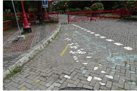
Figure 26 - State 2 - cobblestones (Evenly but not flat paved)
