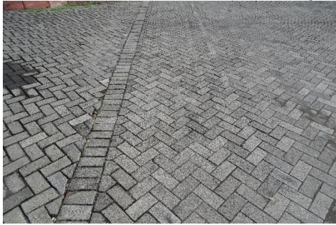
Figure 25 - State 1 - cobblestones (Evenly and flat cobblestones)
