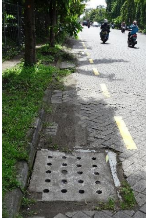
Figure 27 - State 3 - cobblestones (Not evenly paved, with obstacles)
