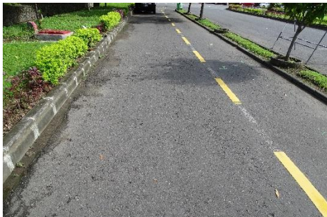
Figure 29 - State 1 - asphalt (Even and flat paved)
