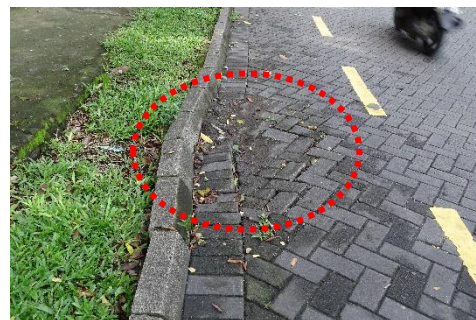
Figure 28 - Sunk cobblestones
