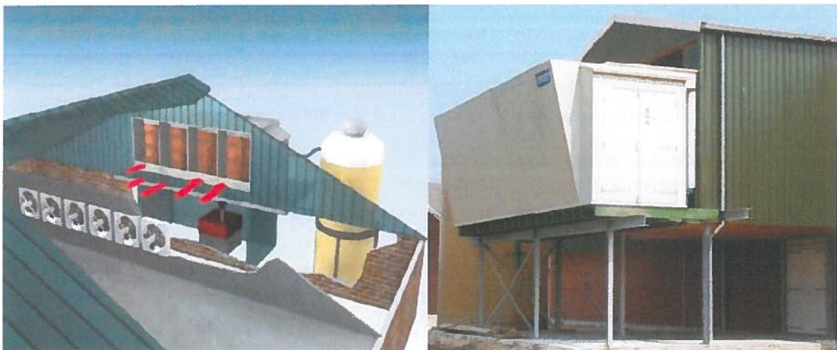
Figure 4-4: Air scrubber used within the agricultural sector
