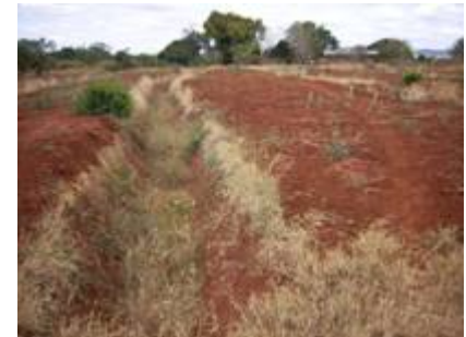
Figure 30. Trenching with grass planting.
