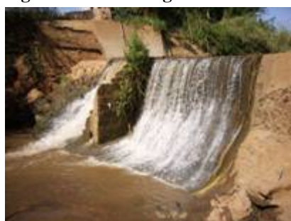
Figure 35. Sand storage dam.
