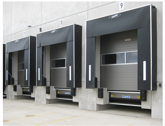
Figure D.1: Docks with a tailgate opening, the opened tailgate fits under the dock. (NovoFerm, 2014)
