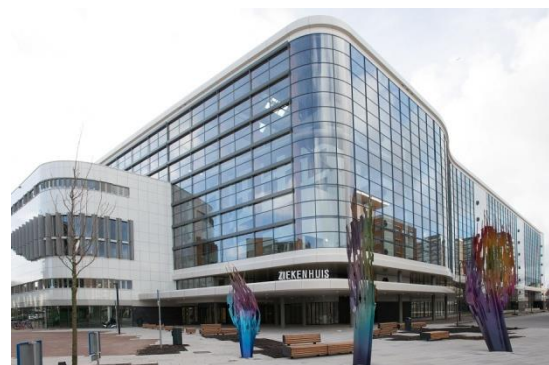
Figure 1.1 The new hospital of MST opened in January 2016
