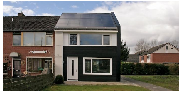
Figure 1. Example of a social renting house renovated to a NoM social renting house. On the left side, the original social renting houses can be seen (Sacon, 2016).
