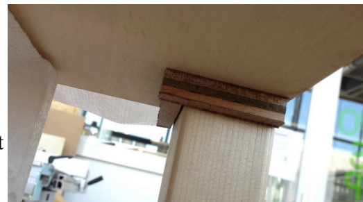
Figure 44: Splints tabletop
