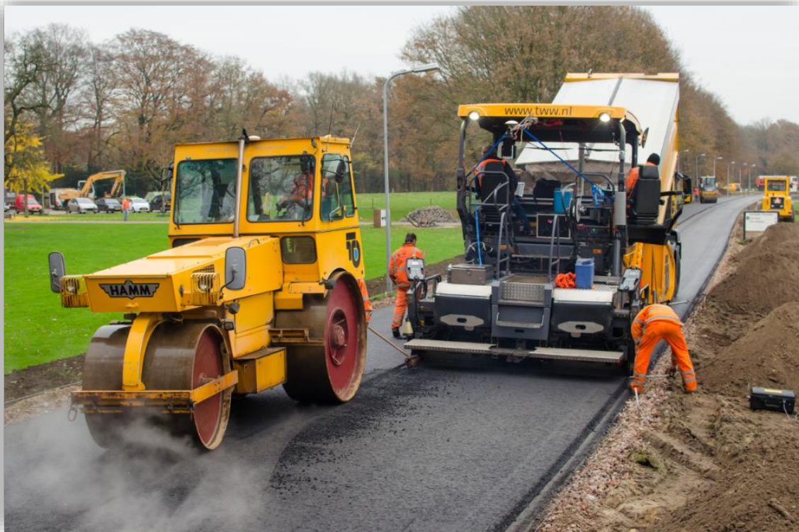
Figure 35: GPS Mounted on a Paver and Roller nov 2014 ASPARi
