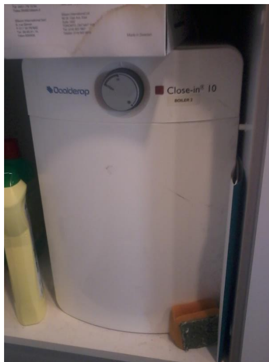
Figuur B2.2: close-in-boiler
