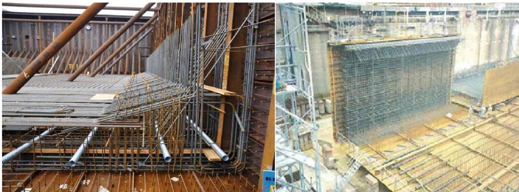
Figure 5 a tunnel section of steel and concrete combined under construction
