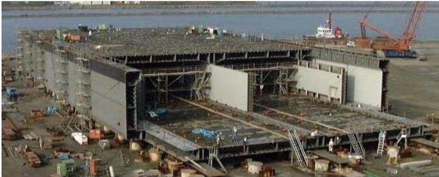
Figure 4 a steel tunnel section
