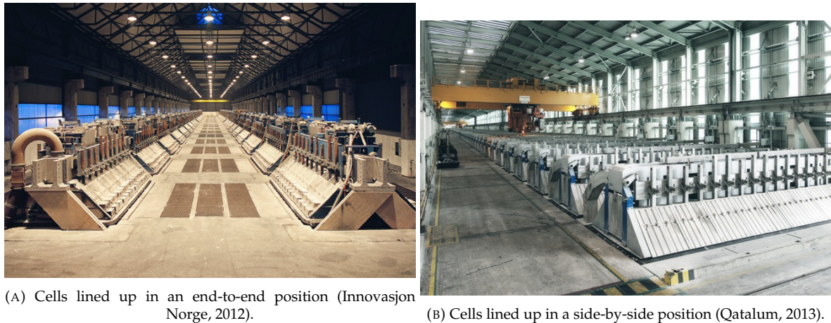
FIGURE 2.6: Different potroom line ups.
