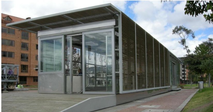
FIGURE 3-8: BICYCLE PARKING BUILDING AT THE 'ALCALÁ' TM STATION (ECONOMÍA EN LA PANADERÍA, 2009)
