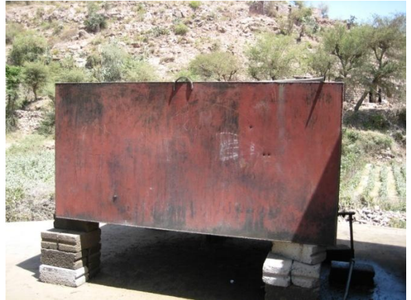
Figure 2: Harbeer 1: Bullet holes in the diesel tank of the water pump Harbeer 1, which has been shot at
