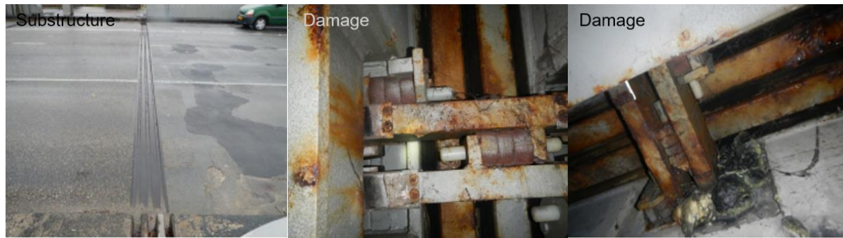
figure 12 - one damage type to the expansion junction
