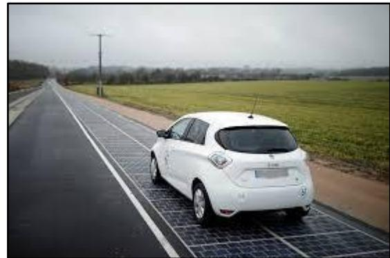
Figure 9: The Wattway solar road from Colas (Materia, 2017)
