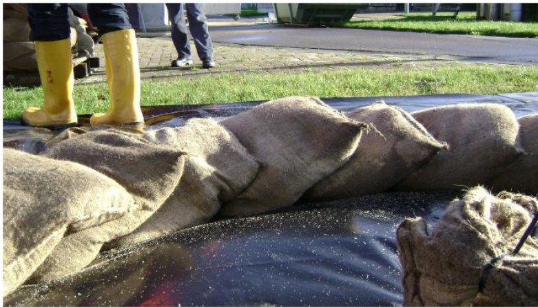
Figure 2.4: Placement of first layer of sandbags (Waterschap Rivierenland, 2017)
