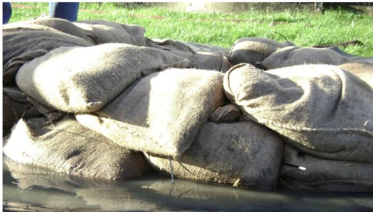
Figure 2.5: placement of additional layers of sandbags (Waterschap Rivierenland, 2017)
