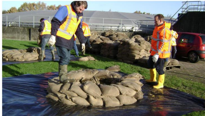
Figure 2.6: Securing the sandbags (Waterschap Rivierenland, 2017)
