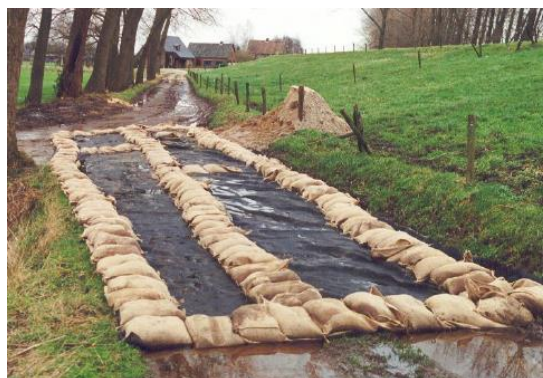
Figure 2.8: Filter construction (Waterschap Rivierenland, 2017)
