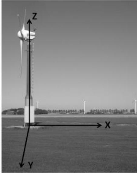
**Figure 2.2:** Coordinate system used in WAKEFARM
