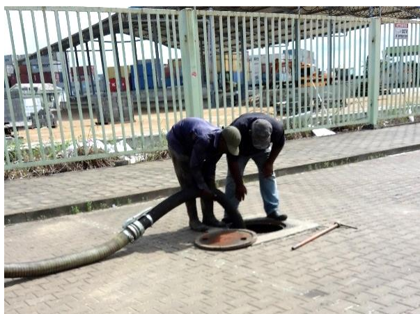
Figure 4.3 - Cleaning of stormwater drainage inspection pits using a gully sucker (source: HBS archive, 2017).
