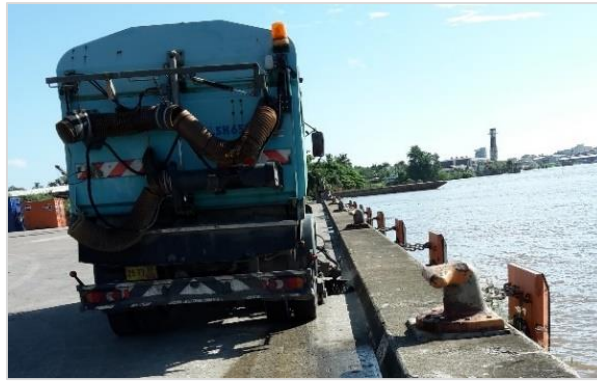
Figure 4.1 - Mechanical cleaning using a vacuum truck (Source: HBS archive, 2016)
