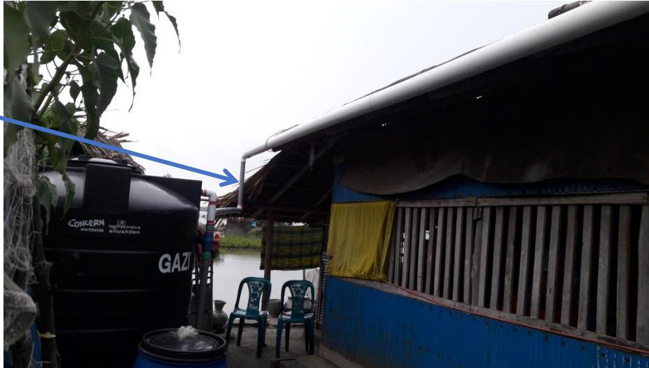
Figure 3.3: Down pipe in rainwater harvesting system (Source: Filed data)
