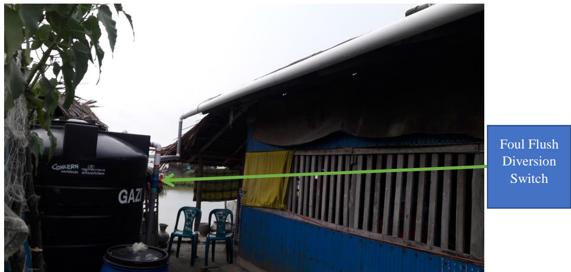
Figure 3.5: Foul Water diversion switch (Source field data)
