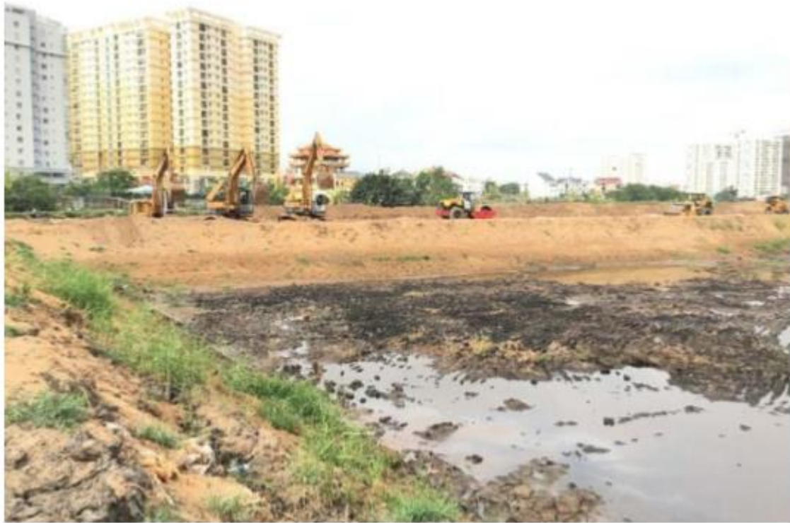
Figure 37. Retention ponds (under construction) near Tan Son Nhat Airport, HCMC
