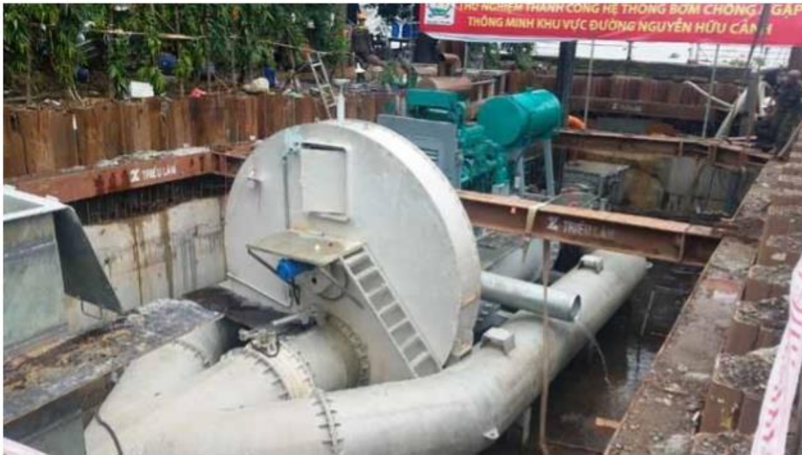
Figure 32. Operating super drainage pump in Nguyen Huu Canh street, HCMC
