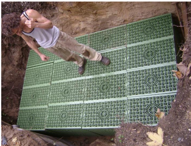
FIGURE 5 - INFILTRATION CRATES (FRITS OGG)
