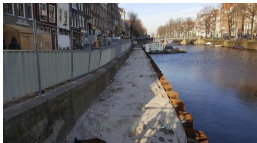
Figure 9: measure to prevent collapsing
