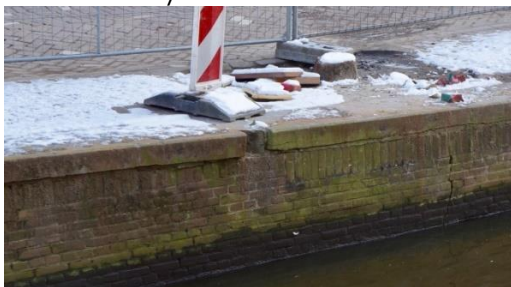
Figure 8: Example of damaged quay wall
