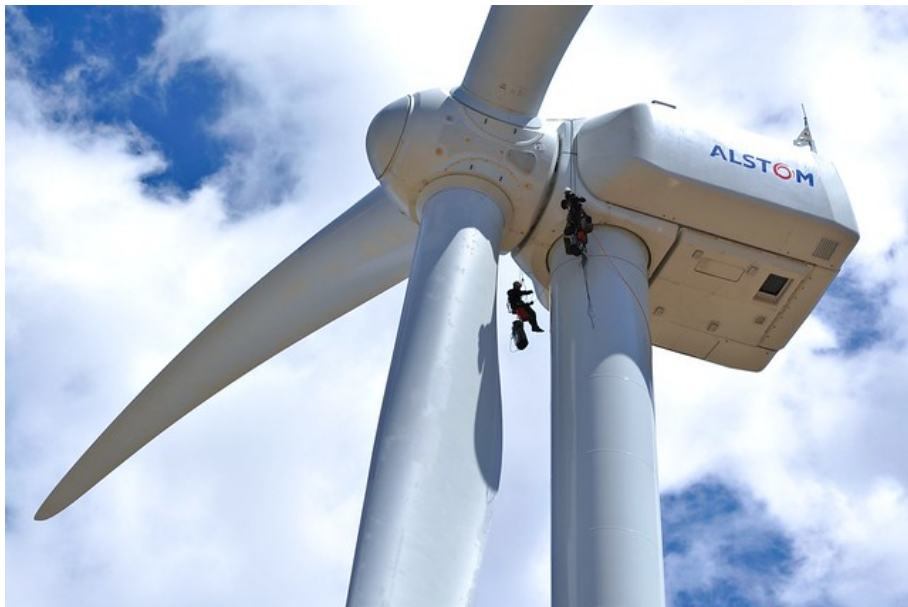
Figure 1.1: Two maintenance engineers using rope access at a wind turbine (Schroeder (2012))
