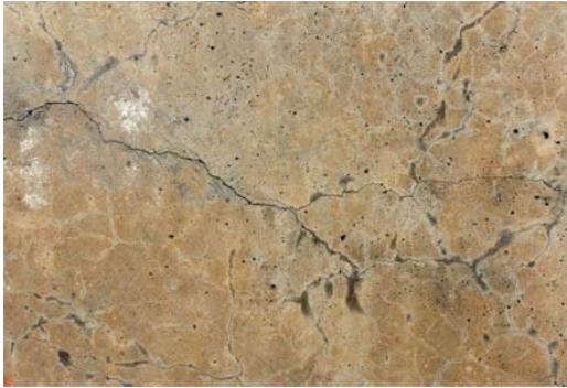
Figure 20: Example of what ASR looks like (Rijkswaterstaat, n.d.)
