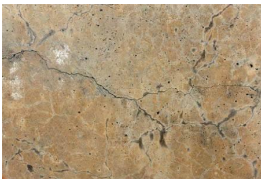
Figure 34: Example of what ASR looks like (Rijkswaterstaat, n.d.)
