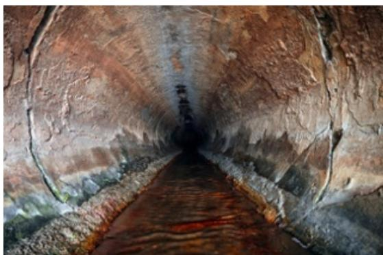
**Figure 2.6:** Corrosion on inner surface of pipe
