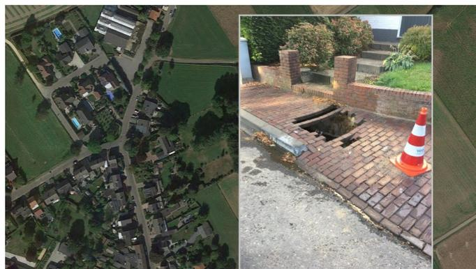
**Figure 2.4:** Accident due to a void
