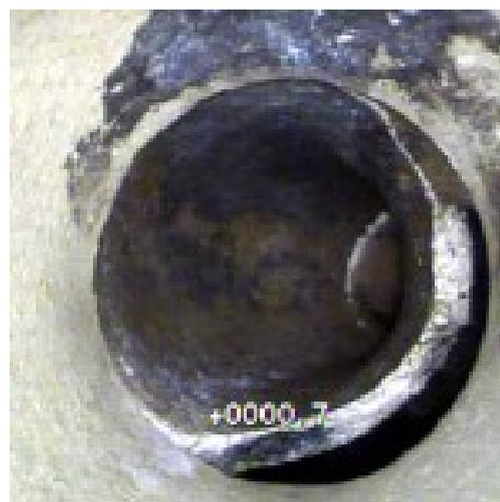
**Figure 2.2:** Joint displacement
