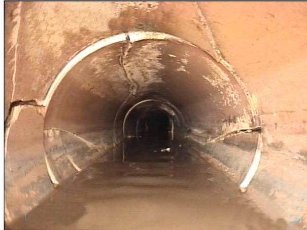
**Figure 2.3:** Crack in a sewer pipe (Tacoma, 2019)
