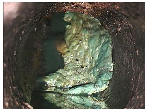
**Figure 2.7:** Encrustation inside the sewer pipe
