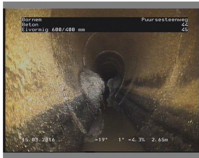
**Figure 2.8:** Root growth inside sewer pipe
