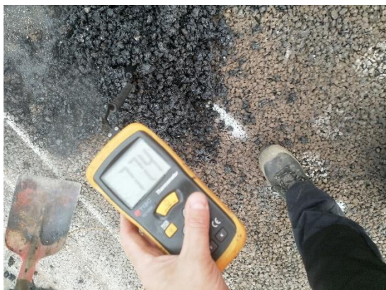
Figure 31: Shovelled heated PA (19-06 11:10)
