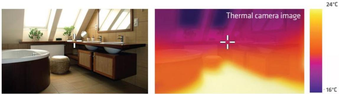
Figure 3-10 An example of underfloor infrared heating system of Heat Décor [57]
