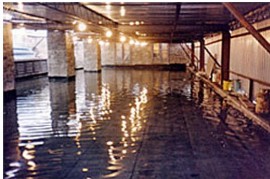
Figure 2: Flood Testing in Progress [3]
