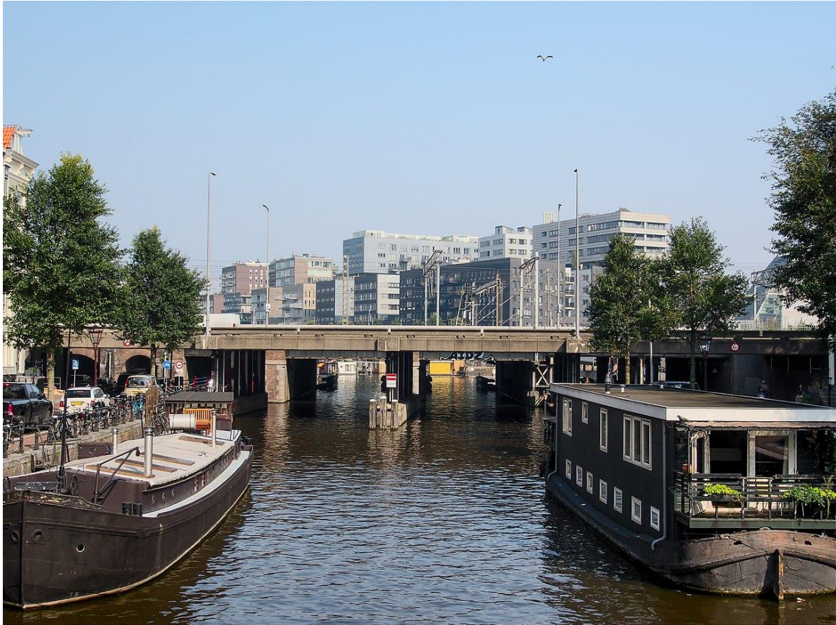
Figure 24 Example scenario: Concrete bridge in Amsterdam
