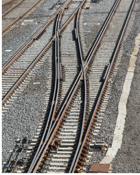
Figure 8: Example of a regular crossover (type 1) - Picture of Wongm's Rail Gallery (WongmsRailGallery, 2014)
