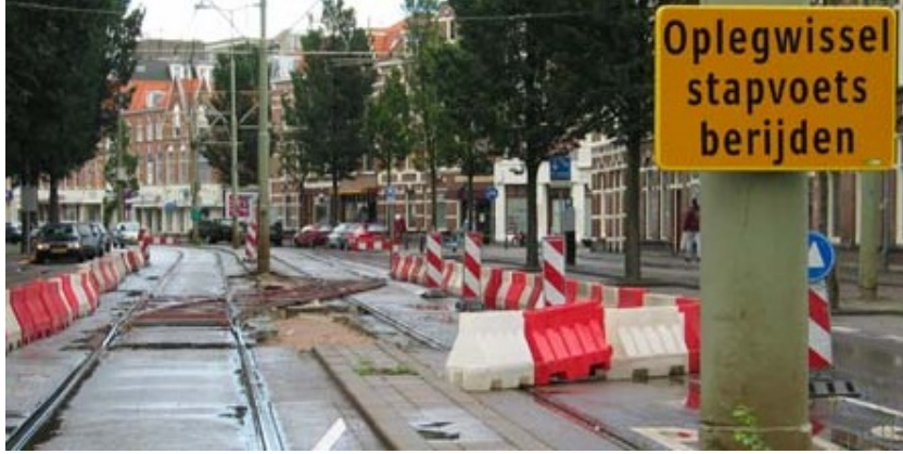
Figure 7: California Switch: a temporary crossover for planned maintenance works. (Picture of DigitaleTram.nl (2005))
