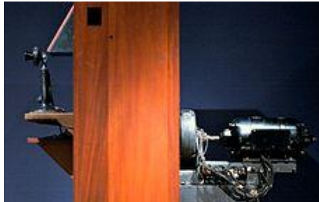
Figure 4 A 1927 Bell Labs videophone prototype
