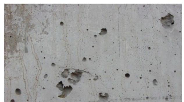
Figure 0-3: Concrete surface voids, source from Google.
