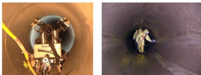
Figure 1-3: Robotic in-pipe-GPR inspection (left) and man entry in-pipe GPR inspection (right), source from the SewerVUE website.
