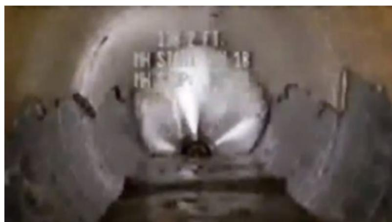
Figure 0-7: Delamination at the pipe bottom, source from Google.
