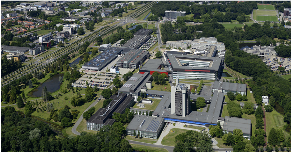
Figure 4.2 Aerial view of the campus
