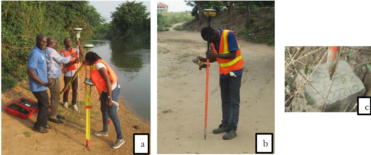
Figure 3-6: GPS Survey work a) Base setup b) Spot height measurement c) Reference benchmark
