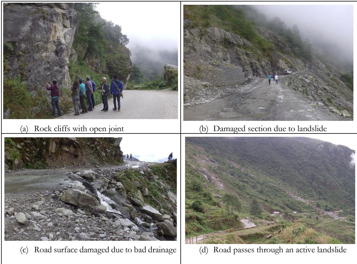
Figure 4.18: Road condition of some segments of Pasang Lhamu Highway after the 2015 earthquake
