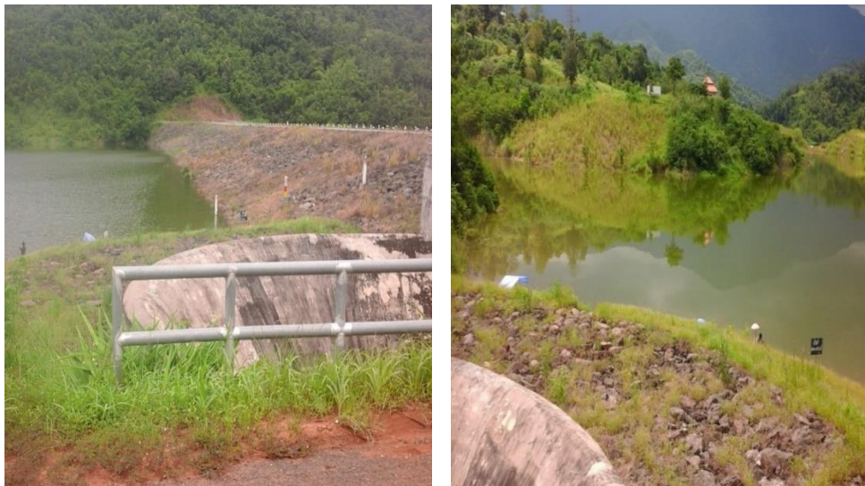
Figure 5.1 Dam for flood control
