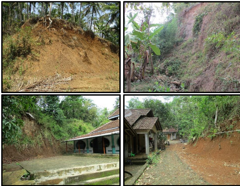
Figure 4-3 Landslide condition in Bompon area
