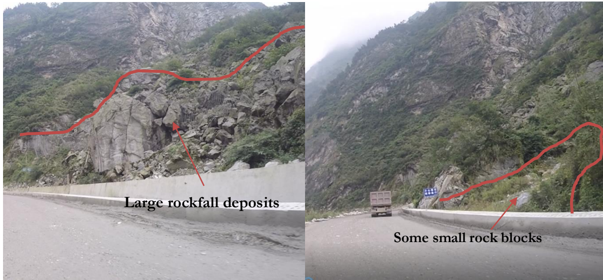
Figure 6.2 Rockfall deposits in section 6.
