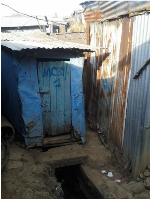
Photo 2a : old toilets being phased out
