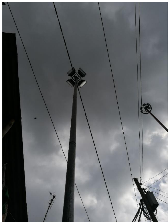
Photo 5b Small floodlight
