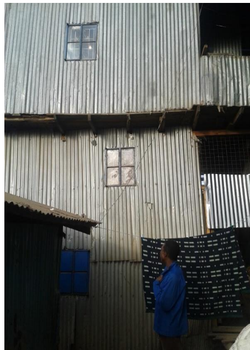
Photo 3b: upward extension to two levels
