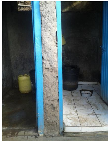
Photo 2b : new toilets being constructed
