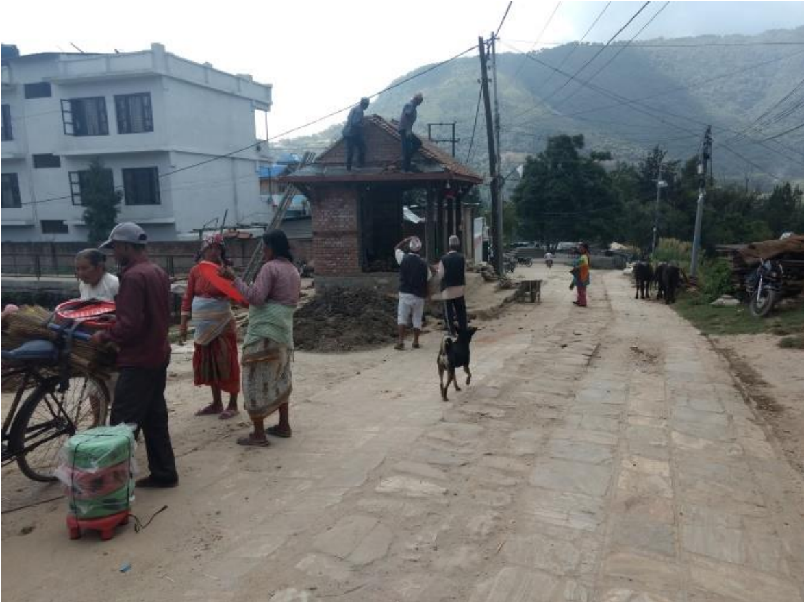
Temple under reconstruction, Khokana
