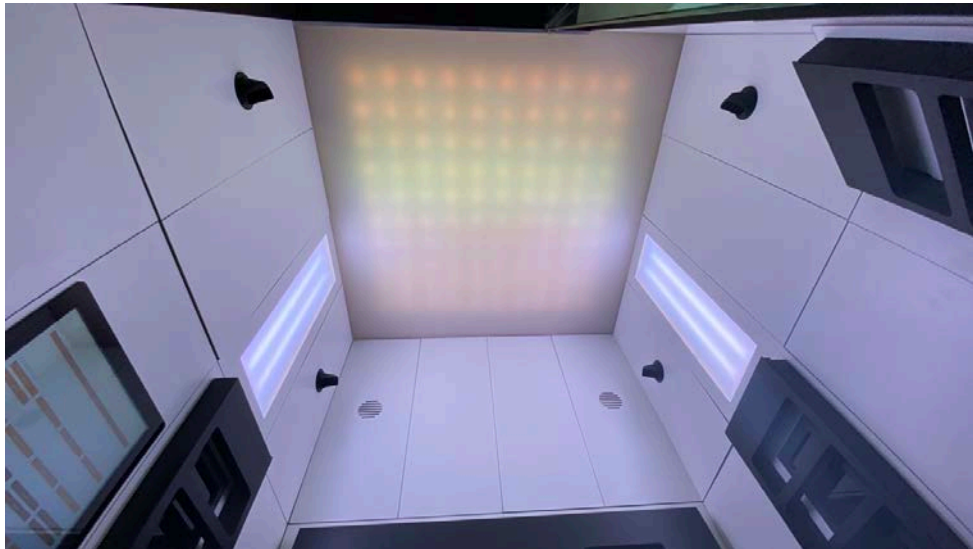
Figure 9-9: The four black angular pieces on sidewalls are ventilator caps.
