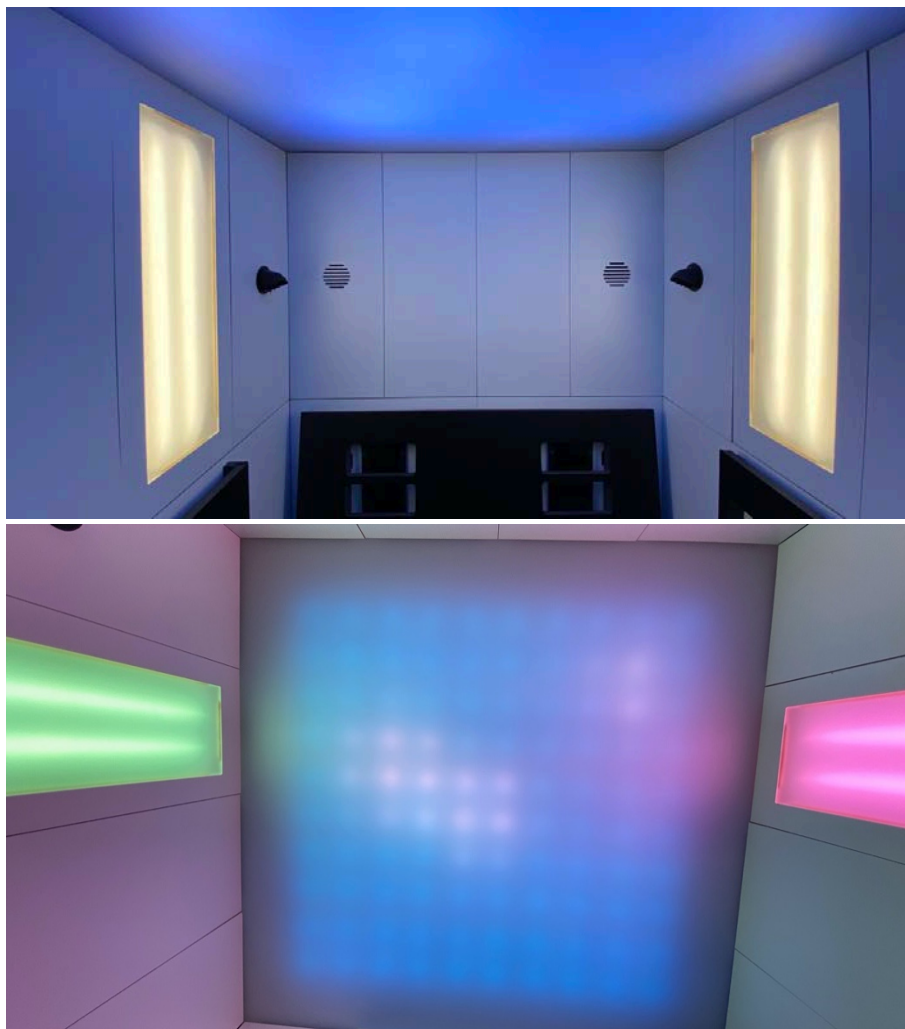
Figure 9-12: The ceiling panel consists of a grid of LEDs and can be animated. The image shows the sun animation pattern.
