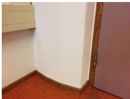
Figure 3- 4 Obstacles at corner in the indoor environment
