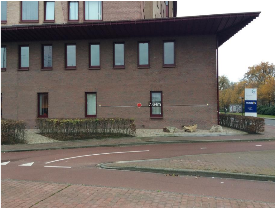
Figure 5.3: Wall facade measurement
