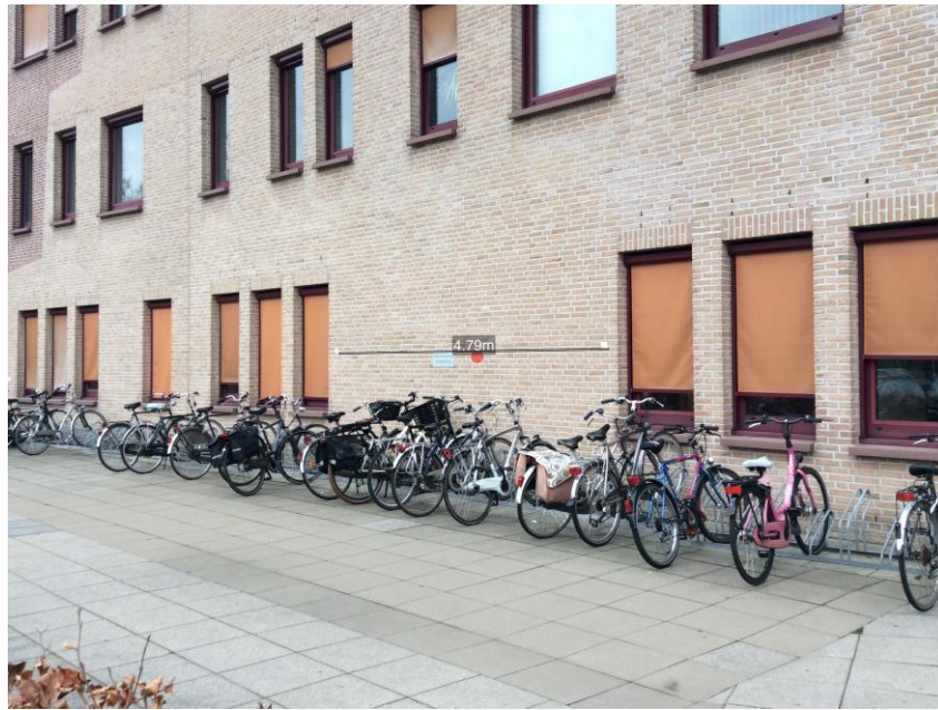
Figure 4.22: Measurement of brick wall
