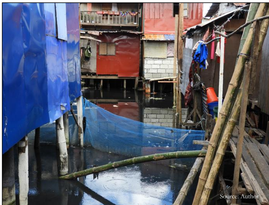
Picture 14: Use of net to prevent solid waste blockage (Cluster 1)
