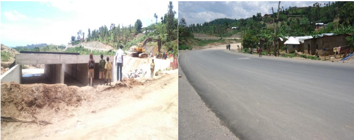
Figure 4-6: Kivu Belt Multinational Road under construction
