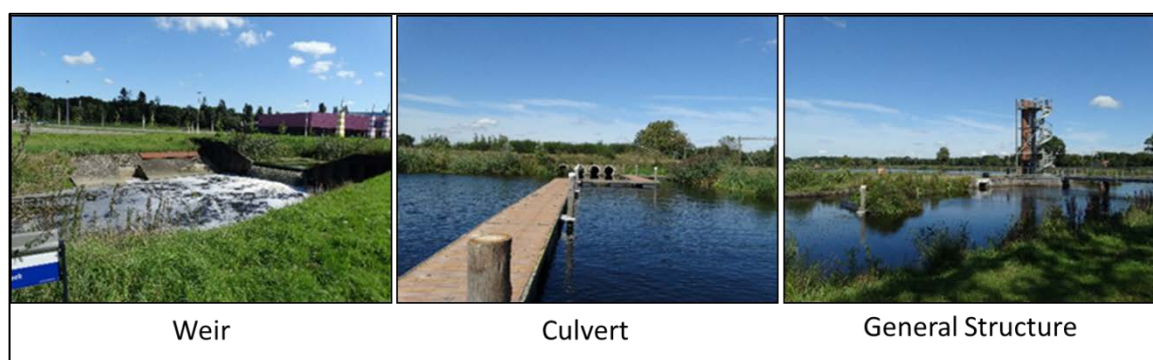
Figure 5 Hydraulic Structures in the Kristalbad
