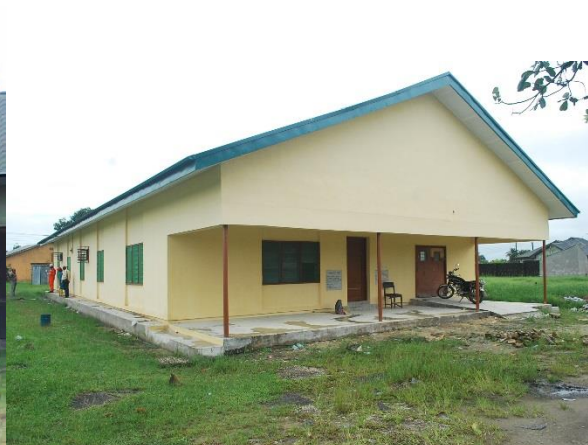
Renovation of Health Center at Ibenu
