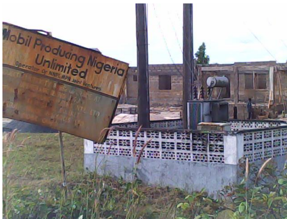
Electricity project at Ibenu
