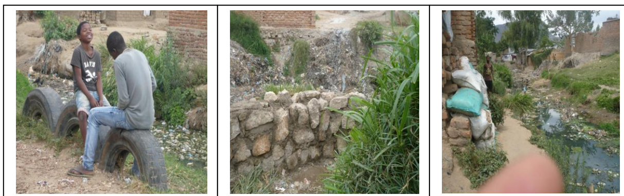
Figure 18: Some observed flood coping strategies (old tires-left; stone embankments-middle; sand bags right)(Source: Author, 2014)
