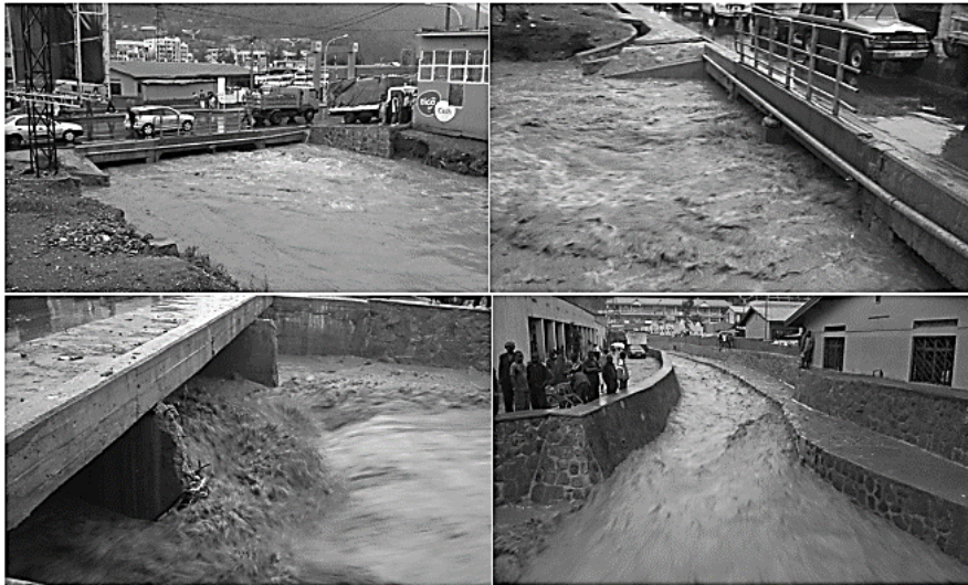
Figure 3.2: Flood waves in the drainage channels photo taken on 2 Oct 2014 during filed wok
